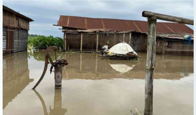
Image 3: Water pumps submerged in water in Sonpura village
